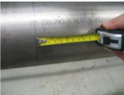
Figure 16: Mark the distance between transducer
